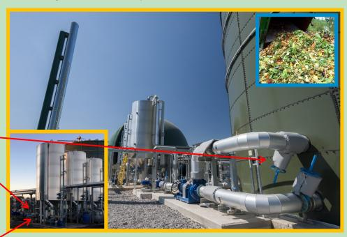
Typically, after shredding/pulping biodegradable feedstocks such as leftover food, crops, sewage and animal waste they are fed into a hydrolysis buffer tank - This tank holds the initial decomposition process, using water to liquefy organic material into slurry. Before the slurry goes into the main digester it must pass through the pasteurisation process for partial sterilization via controlled heating and cooling.
